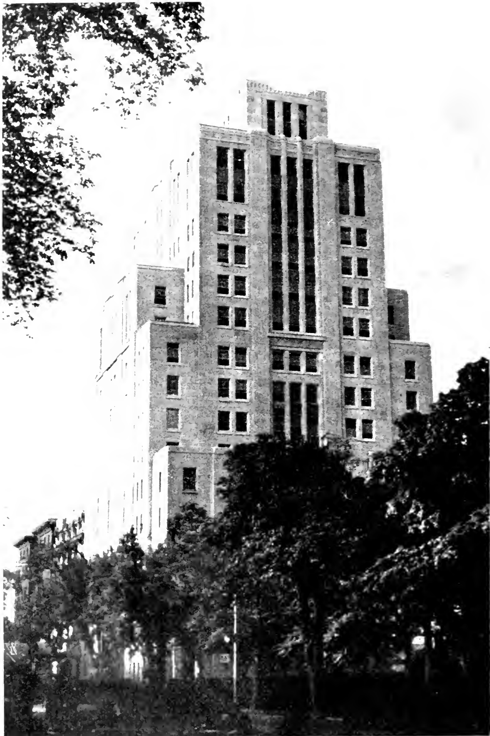
HEAD OFFICE BUILDING - TORONTO Showing addition of ten storeys, completing the new building
